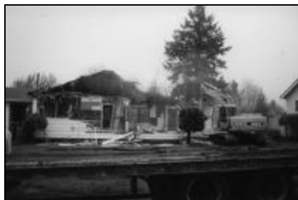
NE 69th Ave—During Demolition
